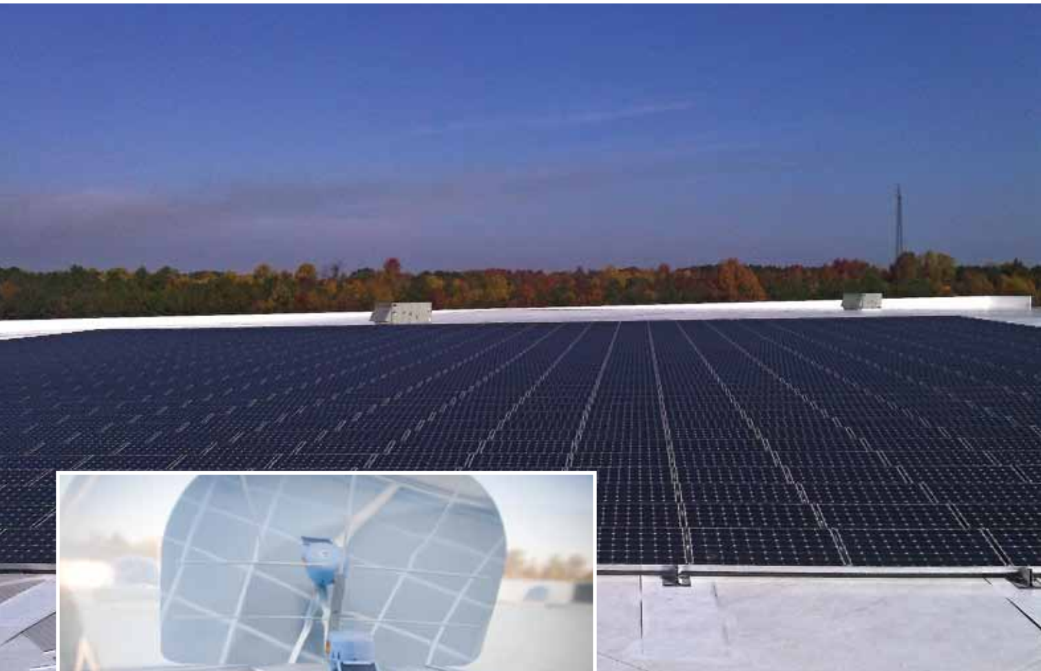
Left: Skylights use solar-powered GPS technology and mirrors to track the sun and deliver natural light, minimizing the need for conventional lighting for the office area. Top: Partial view of four acres of solar panels, estimated to reduce the site's energy consumption by 20 percent.
