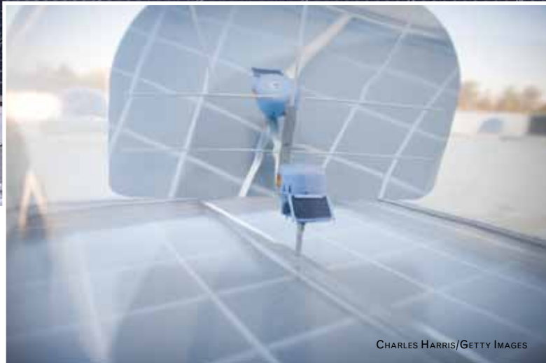
Left: Skylights use solar-powered GPS technology and mirrors to track the sun and deliver natural light, minimizing the need for conventional lighting for the office area. Top: Partial view of four acres of solar panels, estimated to reduce the site's energy consumption by 20 percent.
